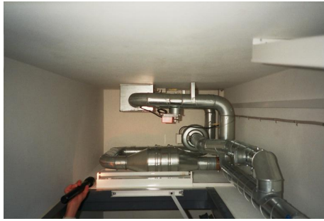
Figure 12: The minimalistic air conditioning apparatus, seen from below. Outside air is blown into the archive only when the building control computer senses that it will push the interior RH in the right direction.
