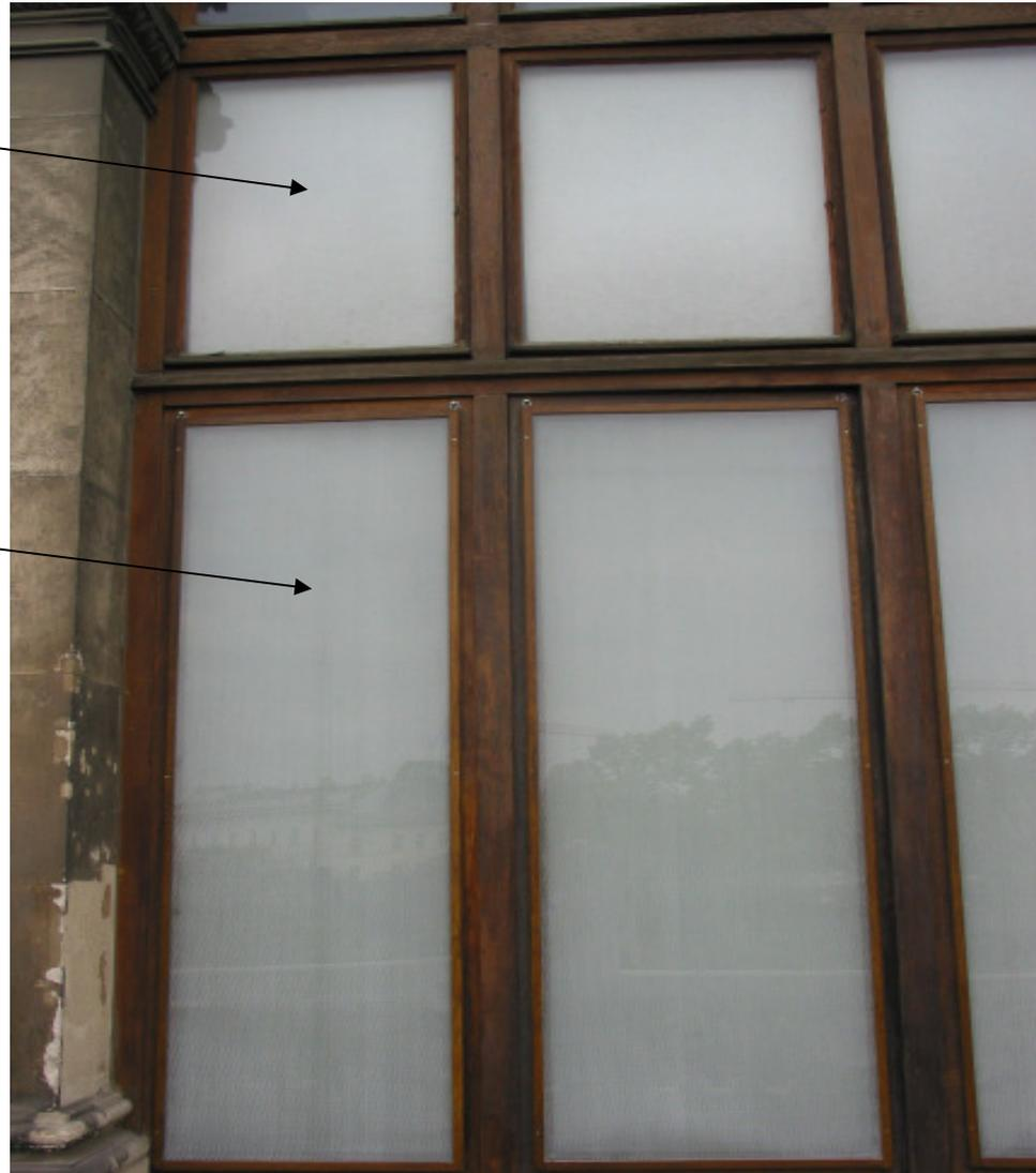
The facade of the Neue Burg with outer shading prototype ...
