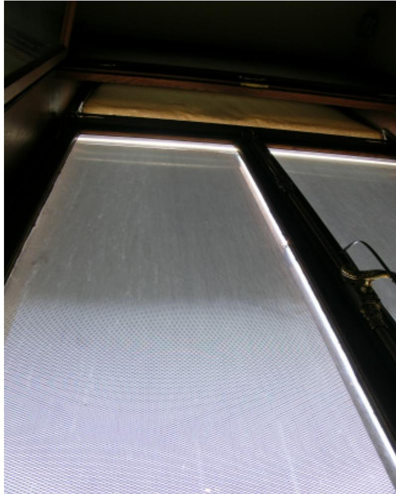
The shading frame is hinged to the outer window frame
