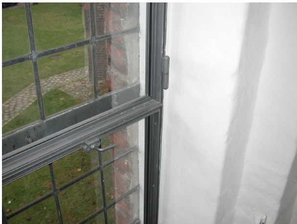
Figure 5. Detail of the windows in Sct. Olai church. The framing for the double glazing was custom designed to fit the original leaded windows. Photo by Poul Klens Larsen
