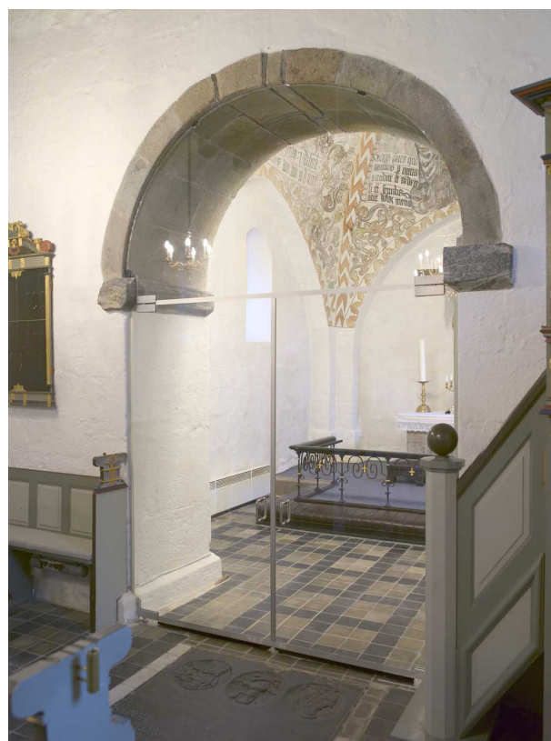
Figure 8. View through the glass door in the chancel arch in Dybe church. The lime painting in the vault is visible in the chancel. The heating elements on the wall below the vault are controlled by a hygrostat to keep the RH at 70-80% all year. Photo by Roberto Fortuna, the National Museum of Denmark.
