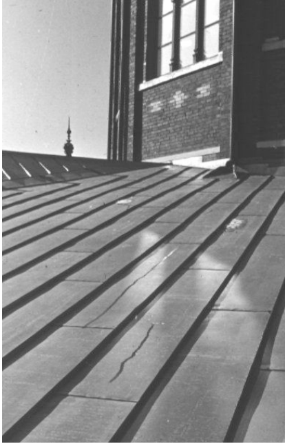
Figure 6.38. Trickles of water emerging onto the roof. The water is distilled from the underlying damp plywood and condenses in periods when the roof skin is cooler than the wood below.
