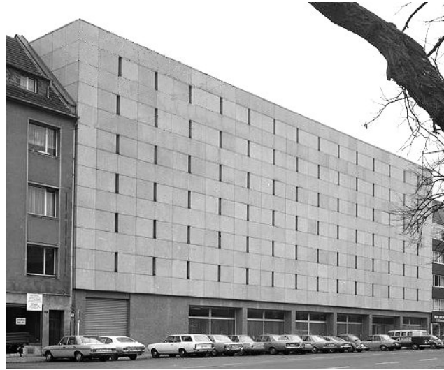
Figure 14: The archive of the city of Cologne. It was built in 1970 on the principle of providing large thermal inertia to prevent the daily cycle of outside temperature from reaching the interior.
