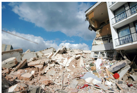
Figure 15: The archive of the city of Cologne after it collapsed into the underground railway excavation in 2009. Photo: Der Spiegel
